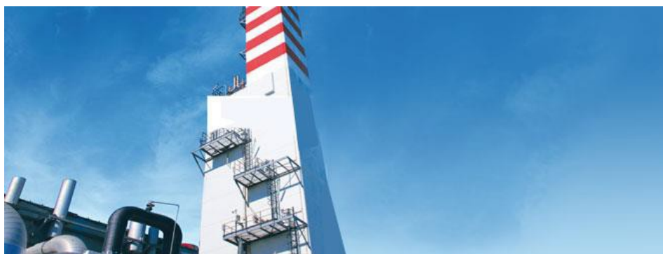
Picture 1a and 1b – CCGT power plant
